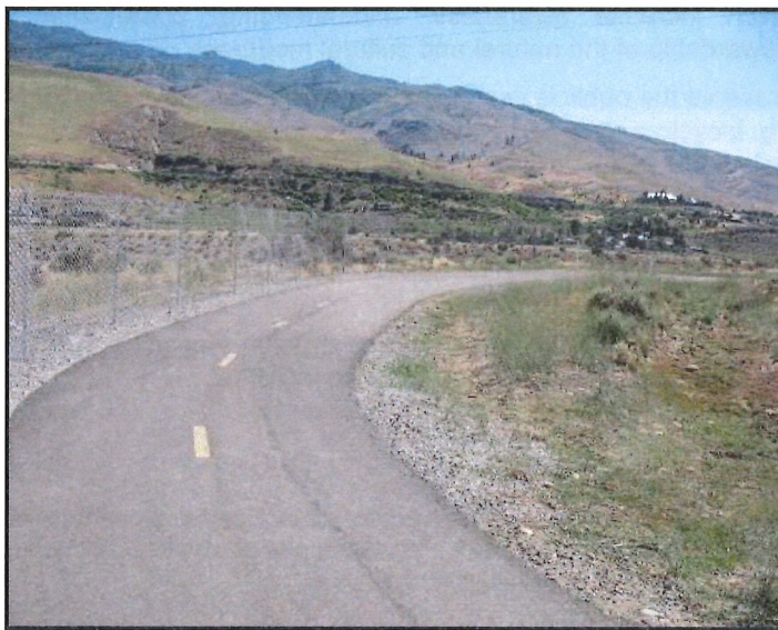
Completed portion of the Tahoe/Pyramid Class 1 bicycle lane near Verdi
