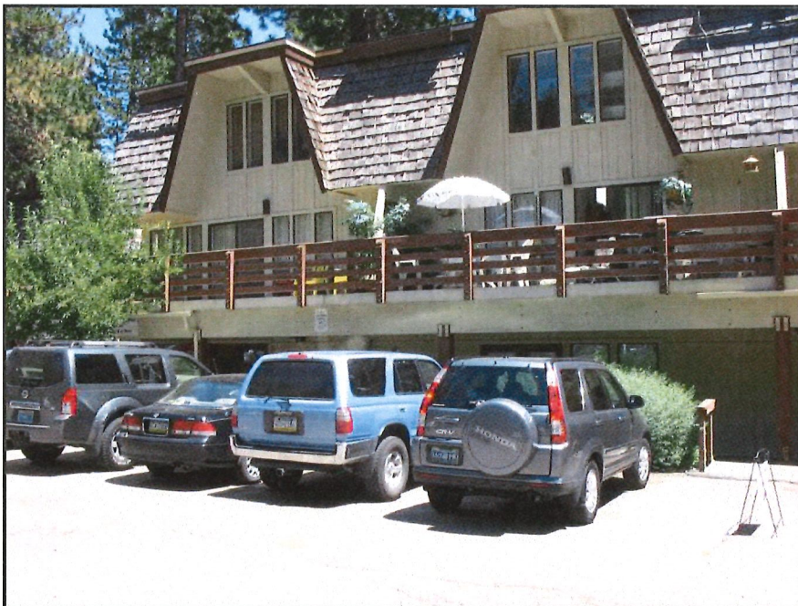
An example of existing unincorporated Washoe County mixed-use located at the Country Club Village development in Incline Village.
